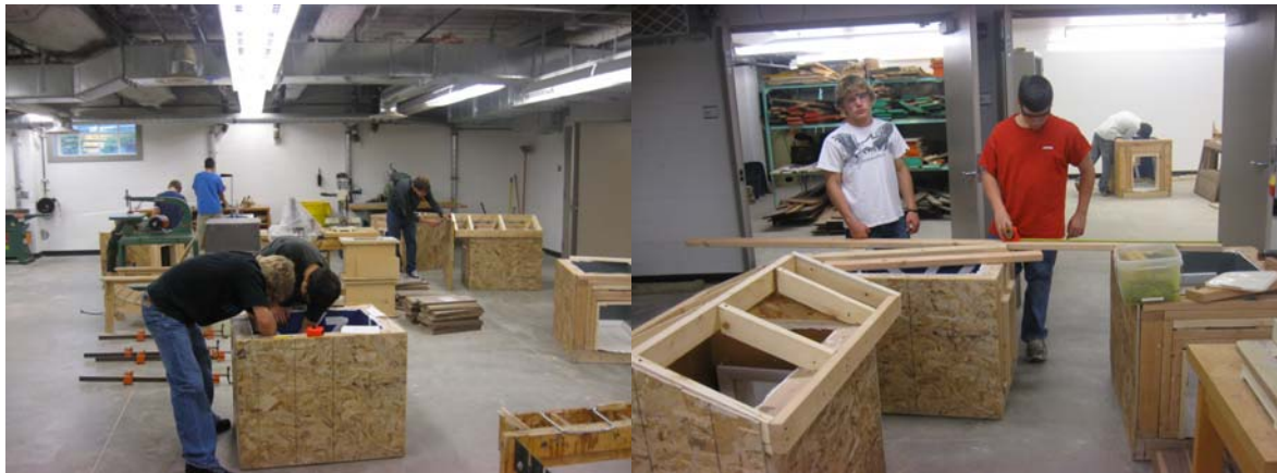
Home Improvement & Design students utilize the new space as they construct a dog house which incorporates framing, roofing, door & window installation, tiling, flooring, and painting.
